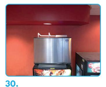
Close the ice machine after turning it on. Plug the ICEZONE into a nearby 100VAC outlet that is not swithed off. The ICEZONE runs 24 hours/day, 7 days per week. Check to make sure the blue light is lit on the top of the ICEZONE.
