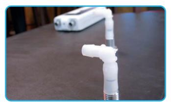
Assemble the supply and return fittings to the 90 degree hose barbs using the 2.5 inch pieces of tubing. *Installer's Tip:* Heating the tubing in hot water eases the installation of the tubing onto the fittings.
