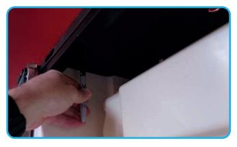
Mark the location for the ICEZONE return fitting. This is the fitting where the plasma will return to the ICEZONE. This should be located on the left side of the top cover (looking at the front of the ice machine). This hole should be spaced off of the interior wall of the ice machine by 1.5 inches. The hole should be spaced from the front frame of the ice machine by 1.5 inches also.
