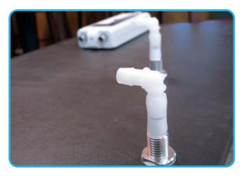
Assemble the supply and return fittings to the 90 degree hose barbs using the 2.5 inch pieces of tubing. *Installer's Tip:* Heating the tubing in hot water eases the installation of the tubing onto the fittings.
