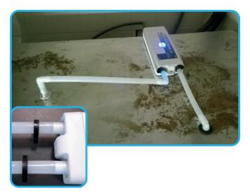
Cut and assemble the remaining supply and return tubing and fittings. Place the handy clamps (black) on the tubing which is placed over the ports on the ICEZONE Unit.
